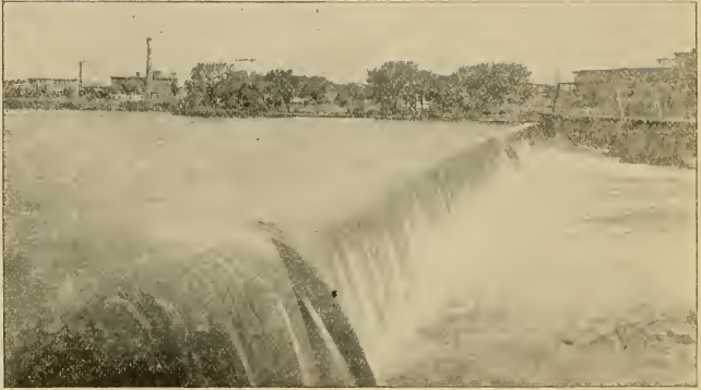
THE LAWRENCE DAM.
